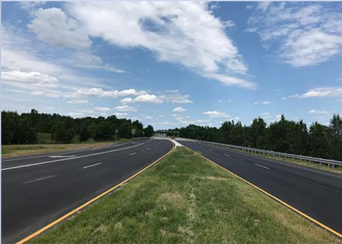
New four-lane configuration of Belmont Ridge Road facing new traffic signal at Dulles Greenway Interchange
